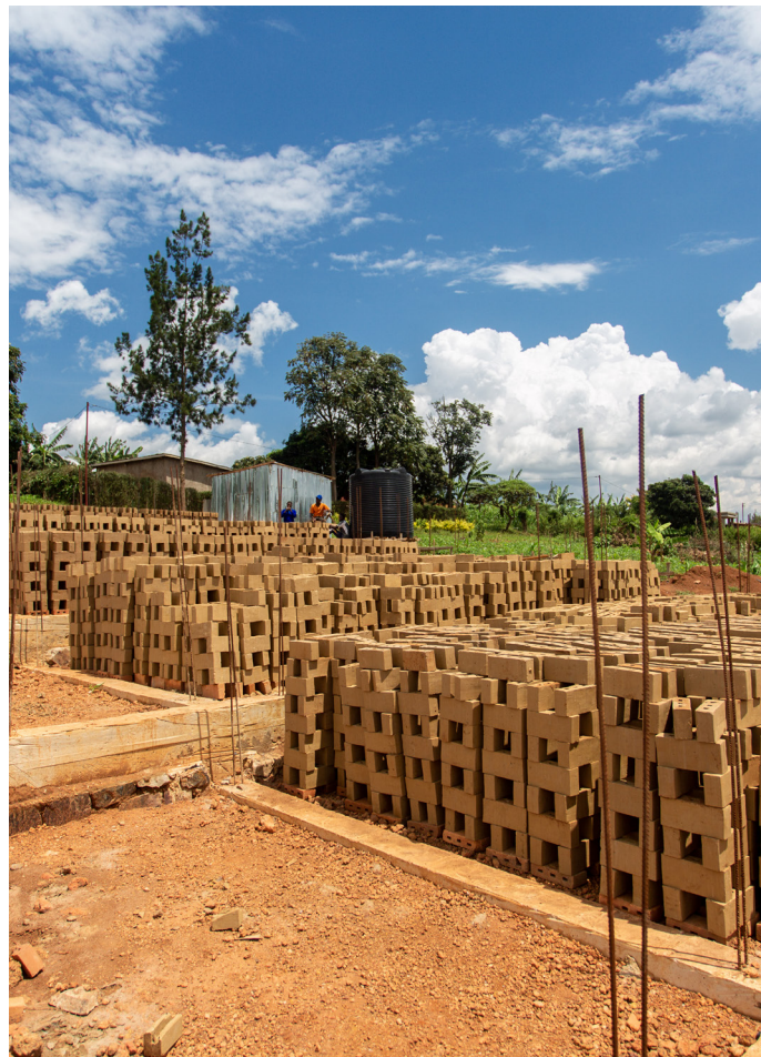
Rectangular piling during secondary drying
